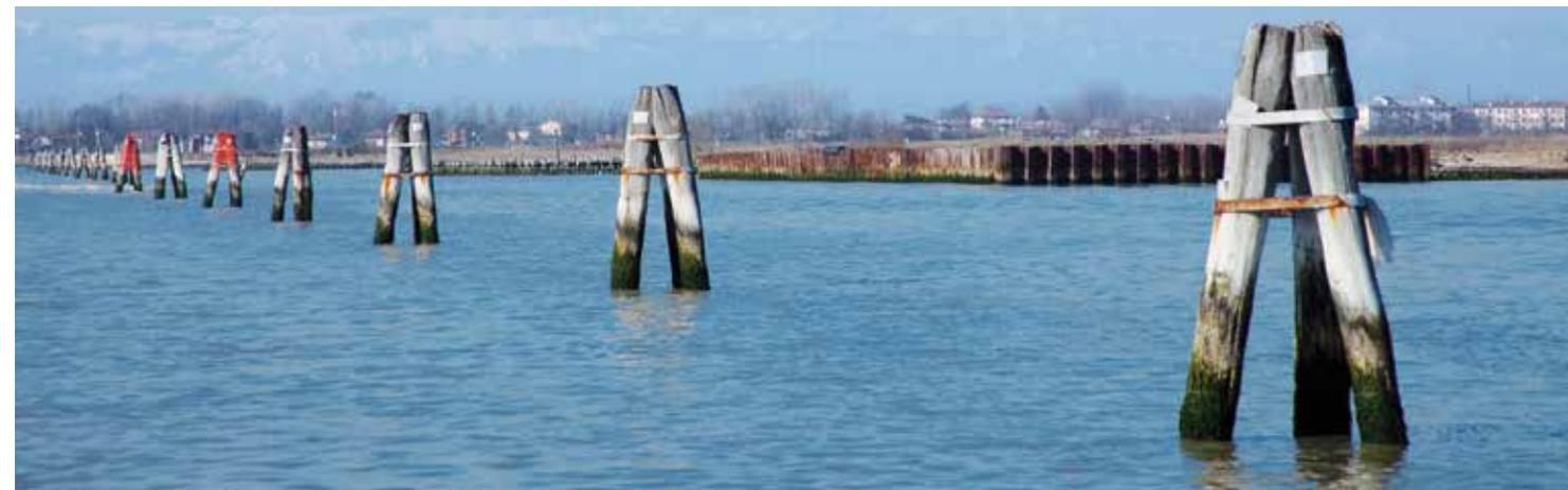
units. As with the pillars of the buildings in Venice, the poles that make up the briccole are predominantly made from European oak, have an average length of from 10 to 15 metres and a diameter between 35 and 50 centimeters. Once unusable they must be replaced, to avoid that, cracking, they may become a danger for navigation. For years the briccole have been made from wood from France and Germany, countries with FSC and PEFC certified forests, whose wood mass is constantly expanding.
